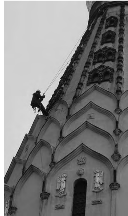
Fig. 7: Work using techniques for rope access and positioning
