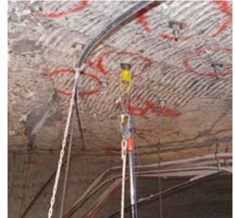
Roofbolts as a connection point for PPE against falls: This idea brought the Award Work - Safety – Health to German mining corporation K+S.
